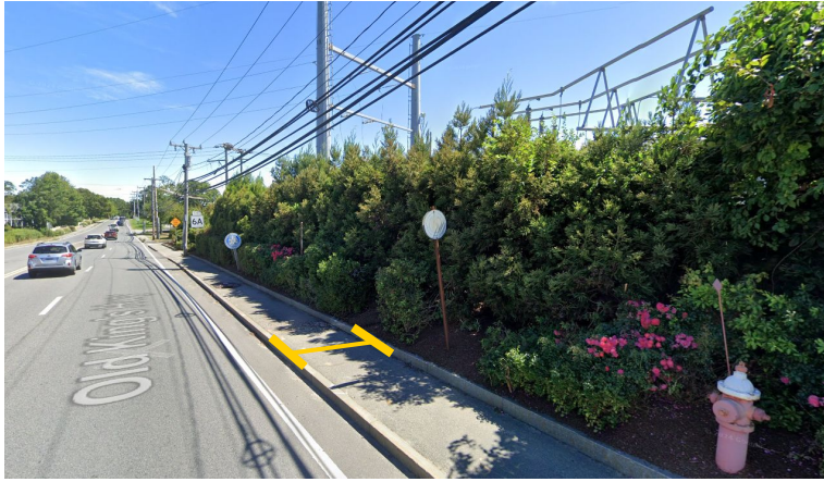
1. Sidewalk Width: 5' Route 6A at Eldredge Park Way Intersection
