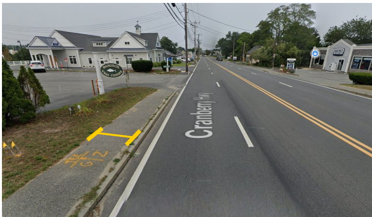
3. Sidewalk Width: 4' Route 6A at Judahs Way
