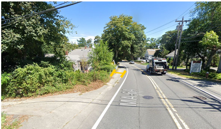
2. Sidewalk Width: 5' Route 6A at Old Tote Road
