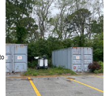
Storage pods at perimeter of site due to lack of storage space and do not provide adequate protection from the elements
