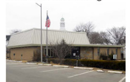
2-Town Hall Annex
