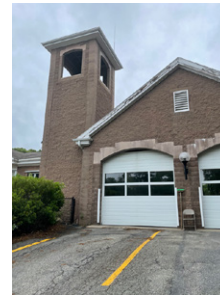
Apparatus bays lack a concrete apron, and asphalt is in poor condition. Precast arch shaped lintels limit effective overall height of doors which limits apparatus selection
