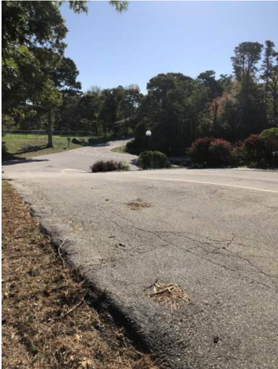
Figure 1.6. Road slope from Apparatus Bay
