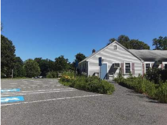
Figure 2.1. Town Hall Annex
