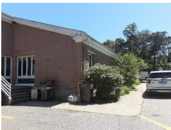
Figure 1.3. East face of building and staff entry
