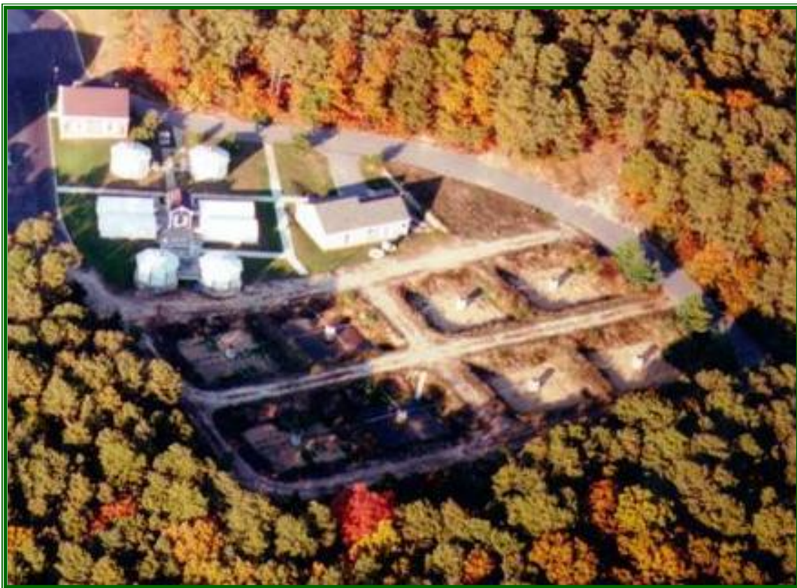
FIGURE 5-2 TRI-TOWN SEPTAGE TREATMENT FACILITY
