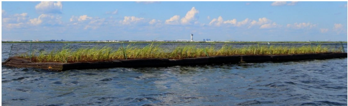
Jamaica Bay Floating Wetland Wave Attenuator
