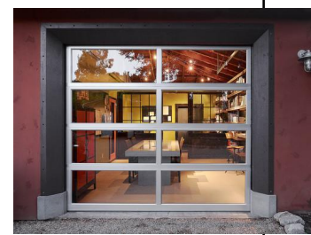
1 OVERHEAD SECTIONAL DOOR, 1 @ 8'-0"x8'-0" 1 @ 16'-0"x8'-0" (ARM-R-LITE 'TITAN' W/ 1" INSULATED GLASS AND ENERGY EFFICIENCY PACKAGE)
